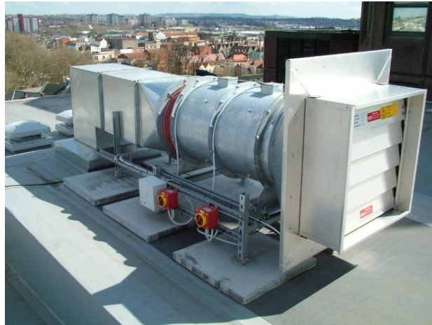
Basic Smoke Control Installation
